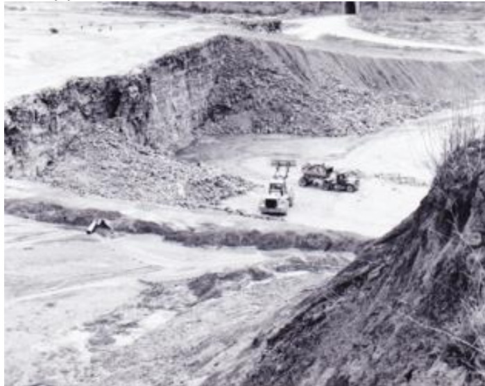
Quarry pit: Lot 18 Con 2 N Oxford - north of CN tracks
