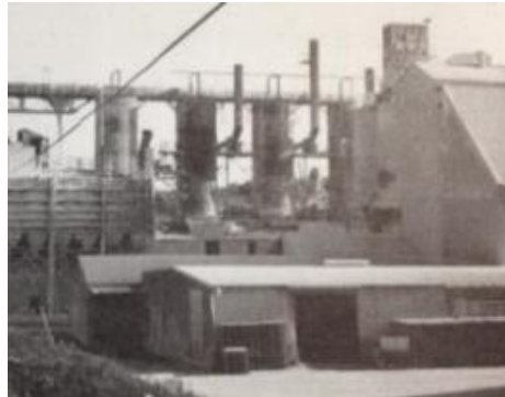
Quarry kiln towers raised by crane
