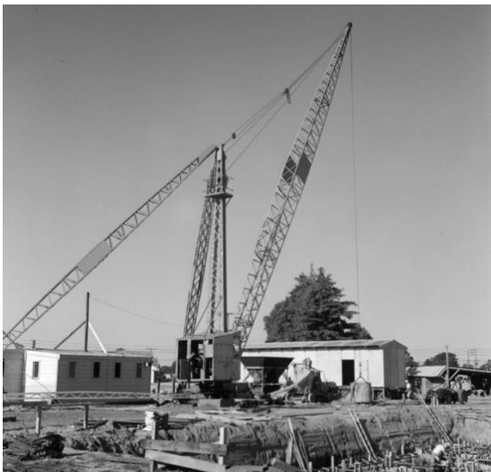
Example of 1950s construction crane.
